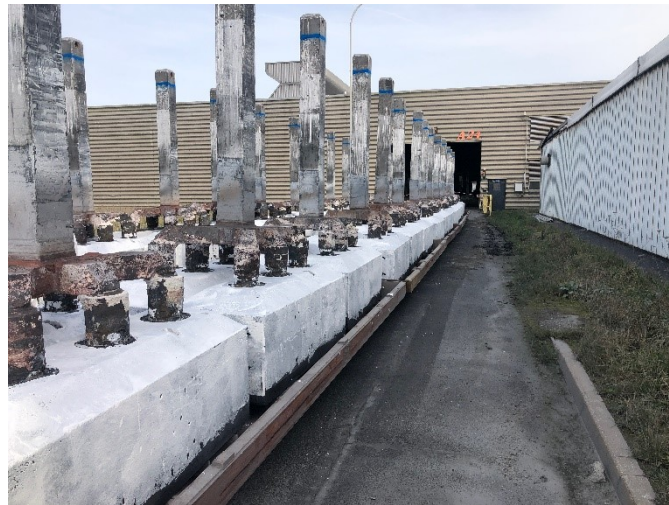
Figure 13. Anodes ready to be used after coating.
